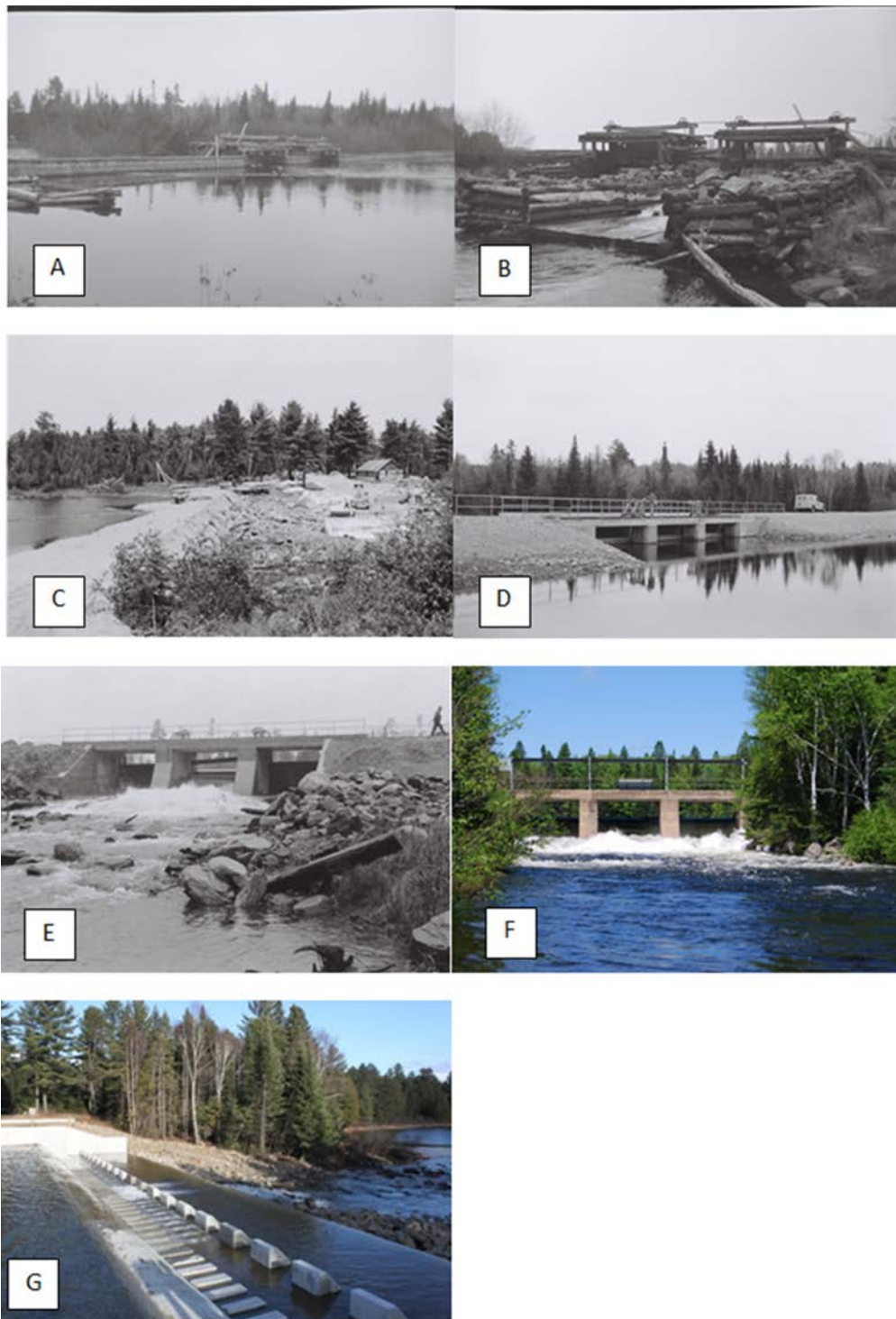
Figure 13. The Annie Bay dam on Lake Opeongo in Algonquin Provincial Park over time: A-B) First dam being used for log transport in the early 20 th century; C) second dam being built in 1955; D-E) second dam operating in 1955; F) second dam in 2011; and G) third ogee (s-shaped) dam operating after construction in 2011. Images C and G have the same perspective.
