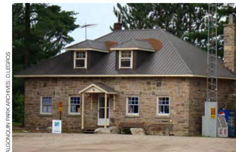
Park Superintendent Frank MacDougall established a Deputy Chief Ranger headquarters at Achray in 1931. Construction of the Stone House to provide an office and accommodation there began in 1933.
